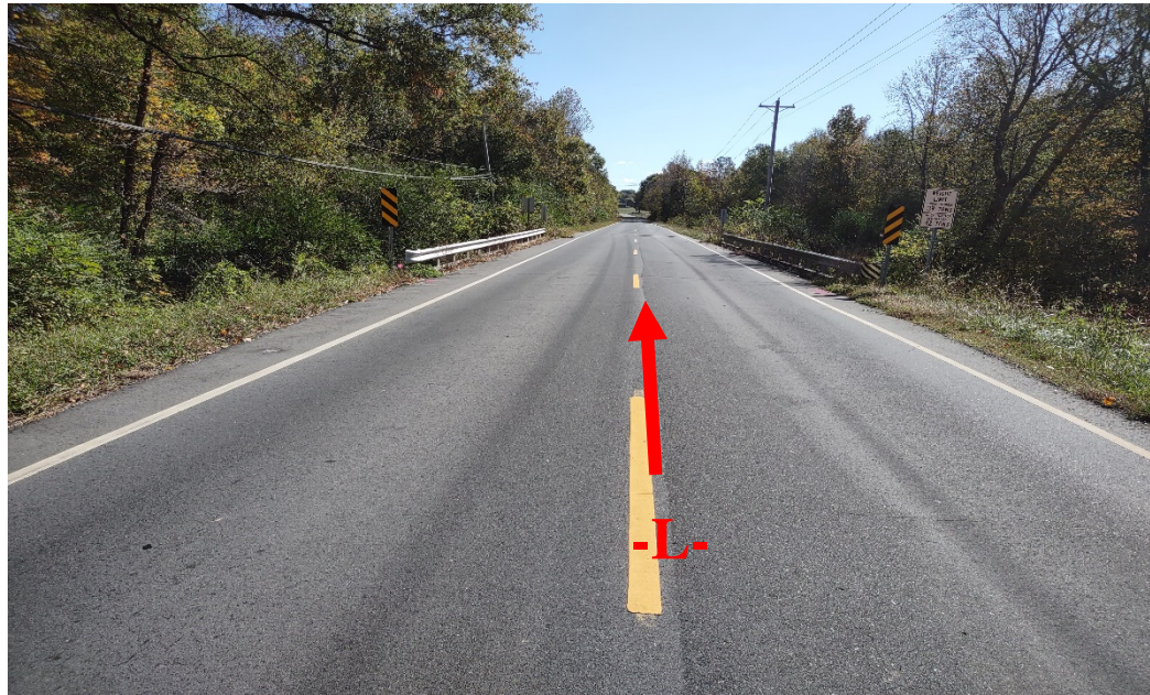
View Along Bridge 246 Looking Upstation
