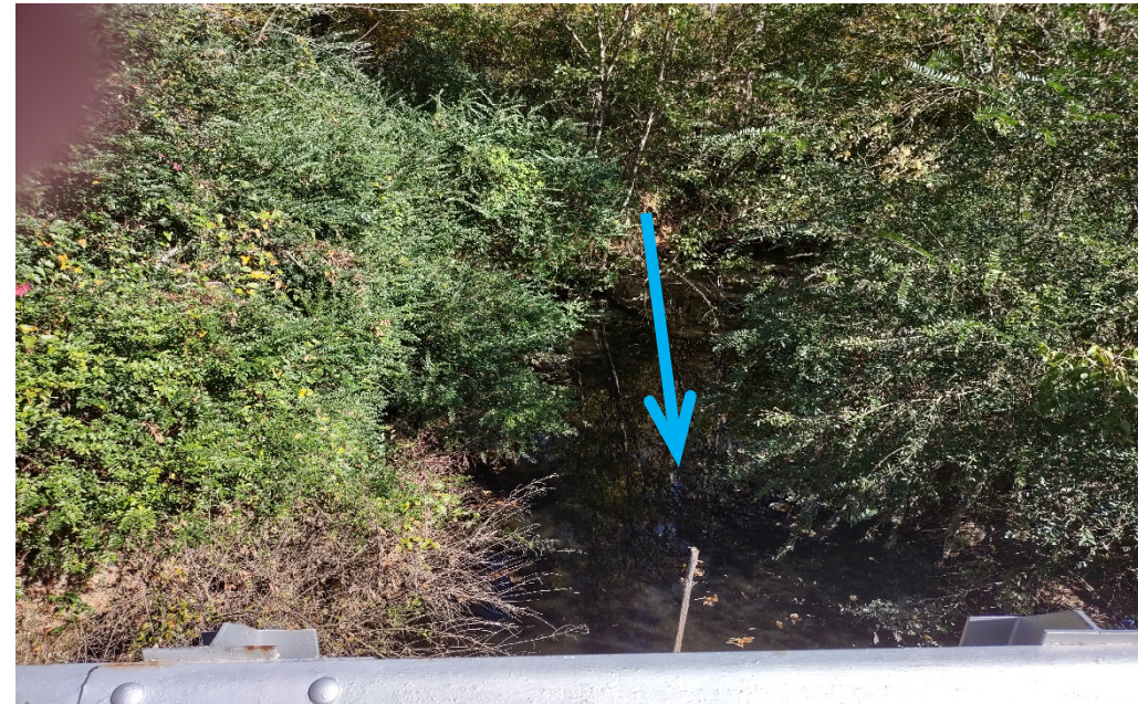
View Looking Upstream from Bridge 246
