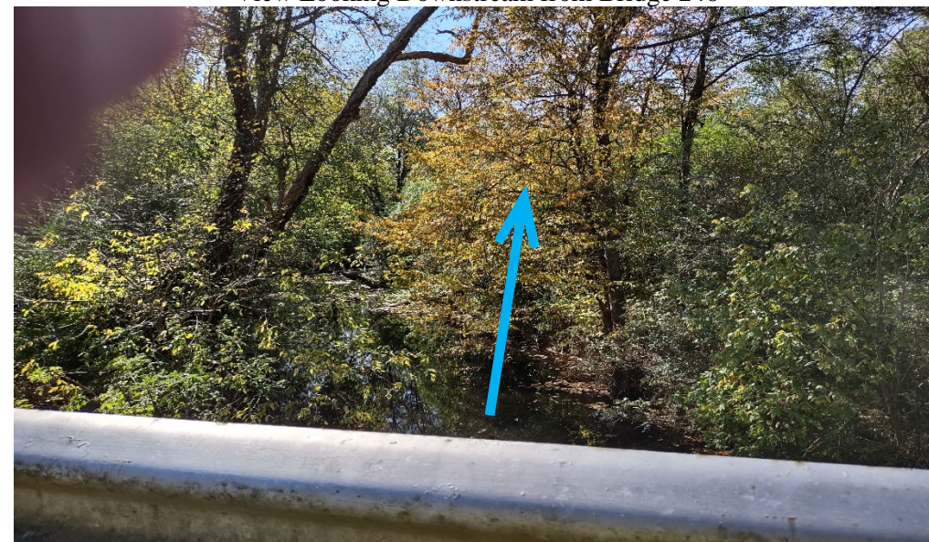
View Looking Downstream from Bridge 246
