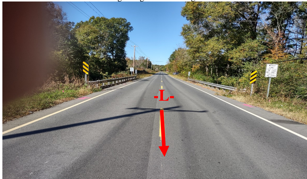
View of Along Bridge 246 Looking Downstation
